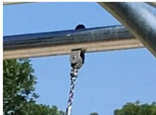
Unique designed swing hangers of stainless steel with anti-twist function. The hangers are attached to the cross beam by a bolt through connection to ensure high durability.
